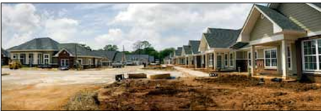
Baldwin Park Senior Village During Construction
